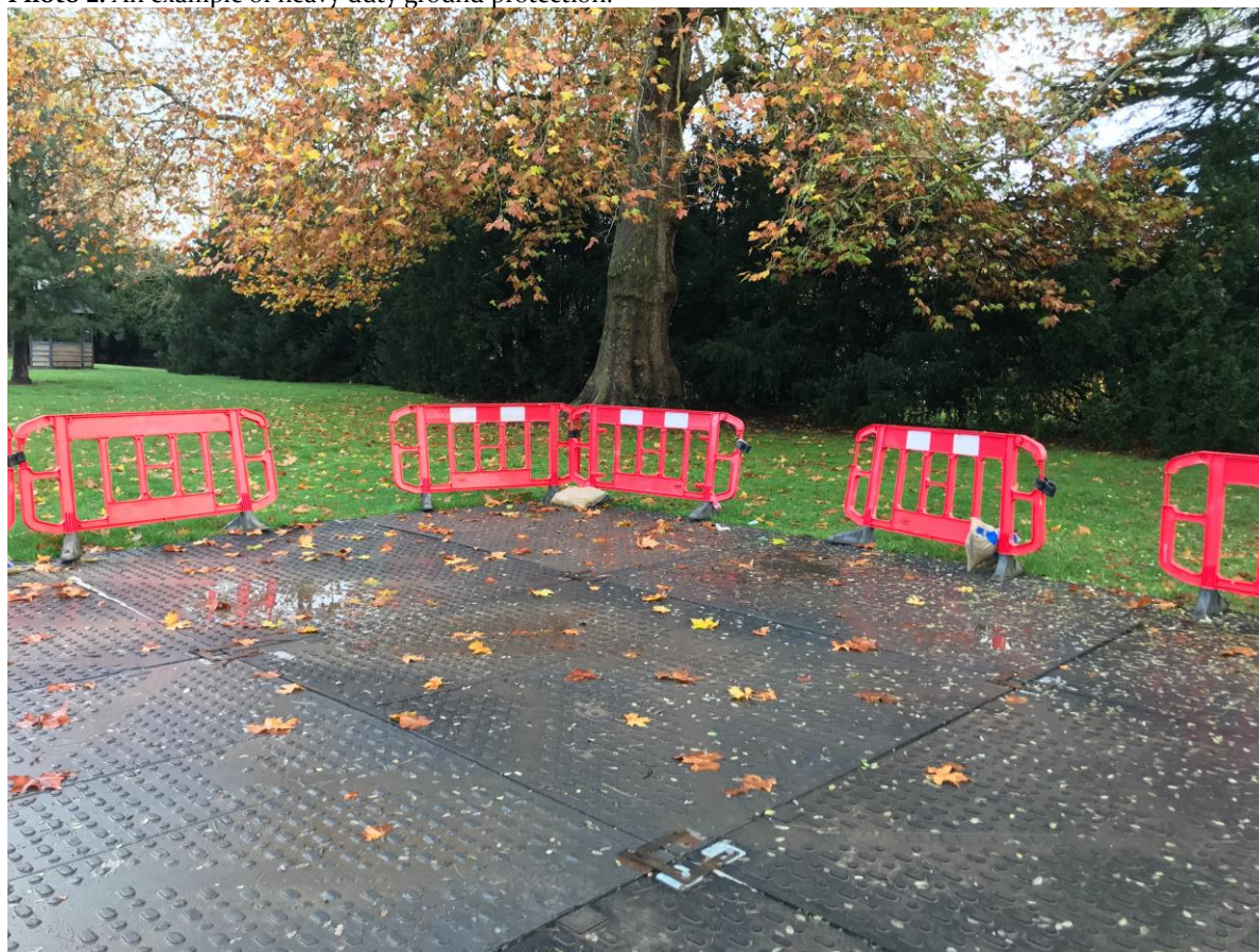
Photo 2. An example of heavy duty ground protection.
