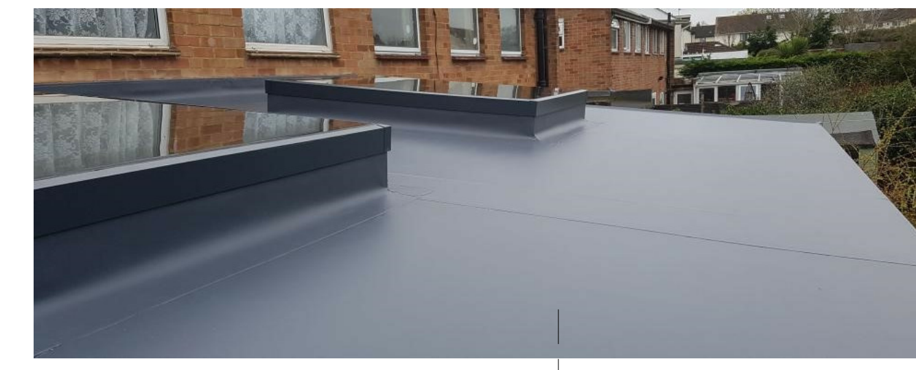
Example photograph of typical roof material finish, inline with existing hotel roof finish
