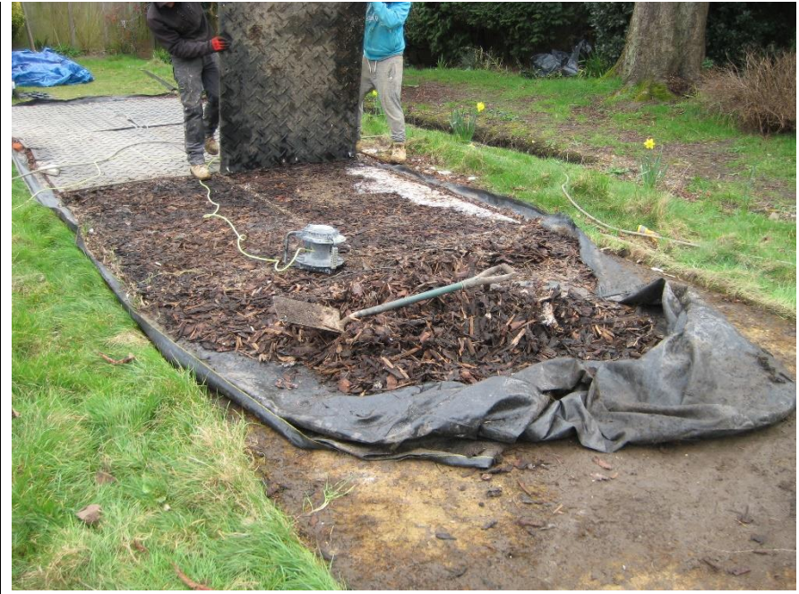
Fig 10 – Temporary ground protection is an effective way of allowing access through the RPA of retained trees. It must be installed prior to any on site activity and maintained for the duration of all works to be effective. Above left Tamla Trees project ground protection in place and above right being removed following the completion of site works. (Note: depending on the length of time it is in place it will adversely affect underlying grass ground cover which will need reseeded/ turfed accordingly).
