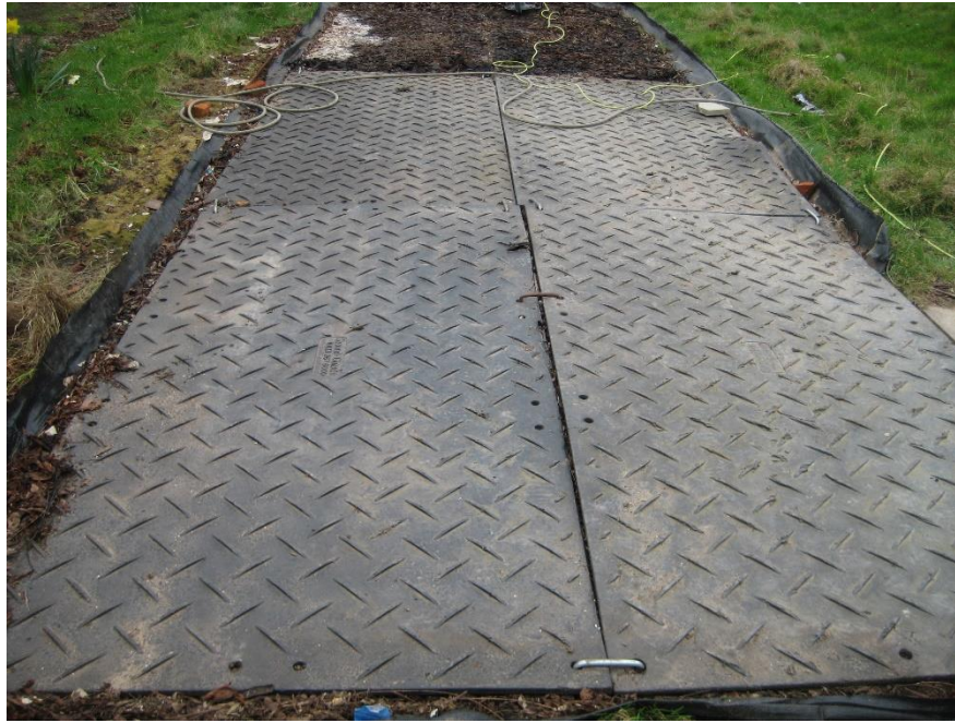
Fig 10 – Temporary ground protection is an effective way of allowing access through the RPA of retained trees. It must be installed prior to any on site activity and maintained for the duration of all works to be effective. Above left Tamla Trees project ground protection in place and above right being removed following the completion of site works. (Note: depending on the length of time it is in place it will adversely affect underlying grass ground cover which will need reseeded/ turfed accordingly).
