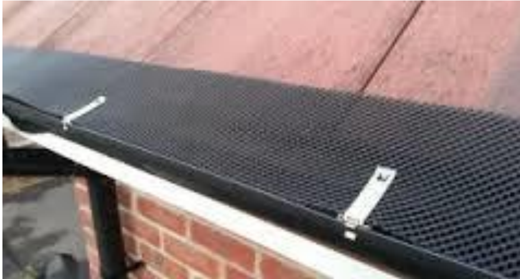
Fig 17 - Suitable gutter guards (2 types shown above) should be fitted to ensure that leaf drop from adjacent trees does not block new guttering leading to potential pressure for tree works.
