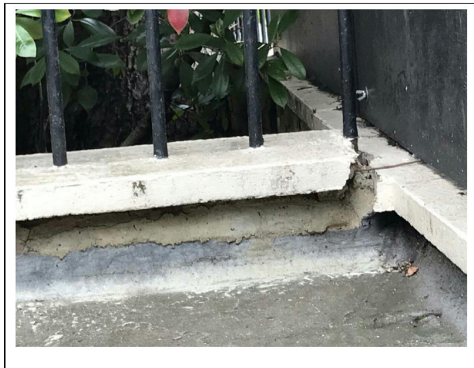
View of crack displacement
