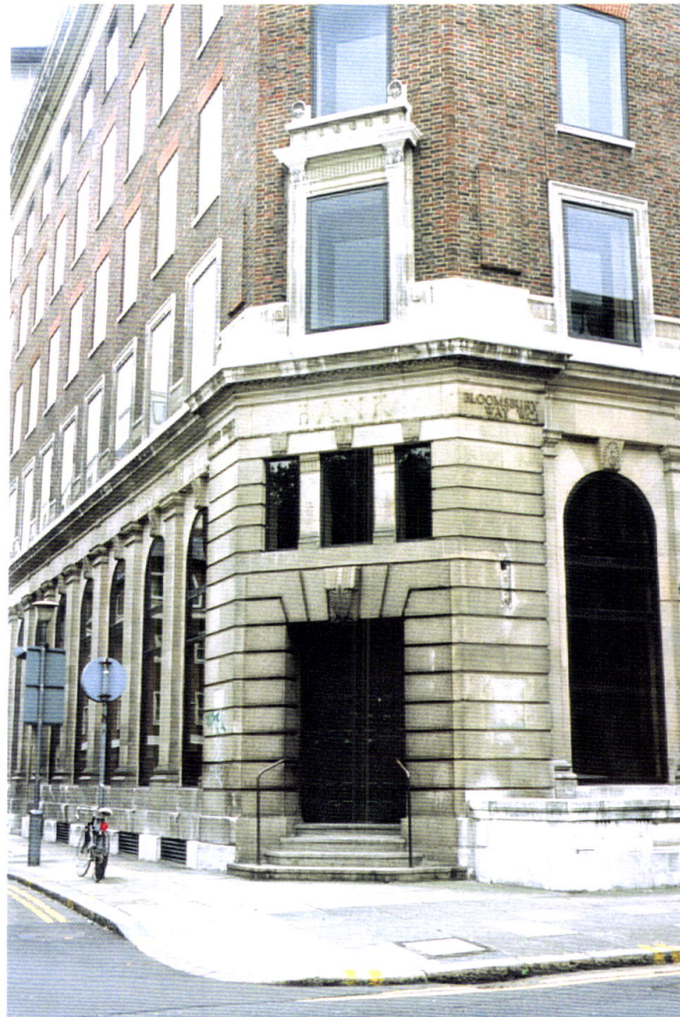
NORTH EAST ELEVATION (Bank Door to be removed and replaced with window to match)
