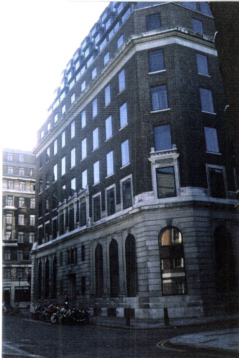
SOUTH ELEVATION (Extra Service door to be added adjacent to existing back entrance)
