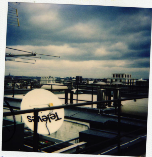
15-19 BLOOMSBURY WAY view from dish location across roof to opposite corner
