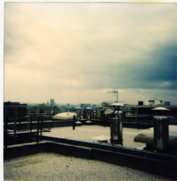
15-19 BLOOMSBURY WAY view towards dish location across roof from opposite corner.
