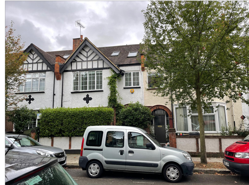
PHOTOGRAPH OF FRONT ELEVATION
