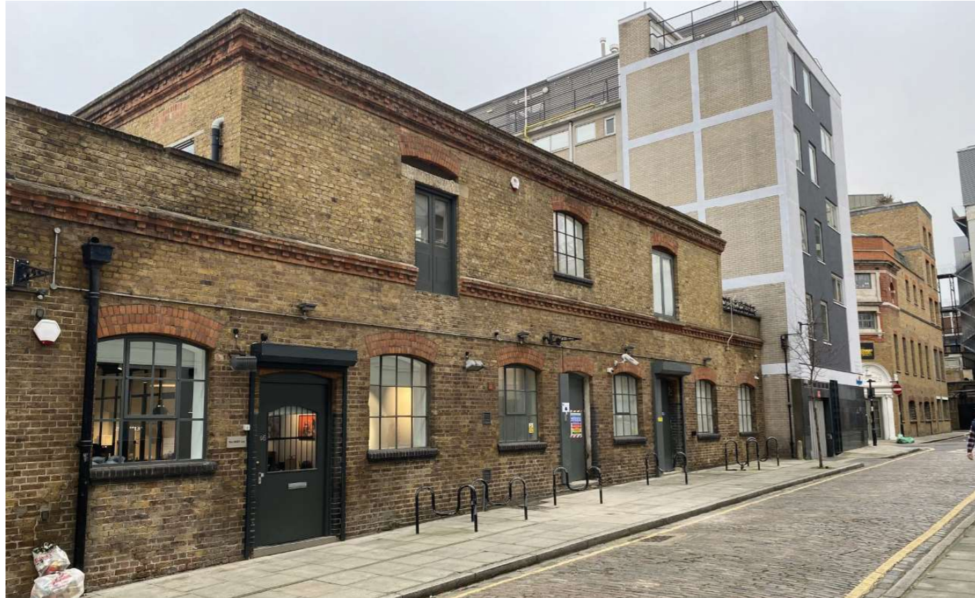
Existing Wicklow Street View
