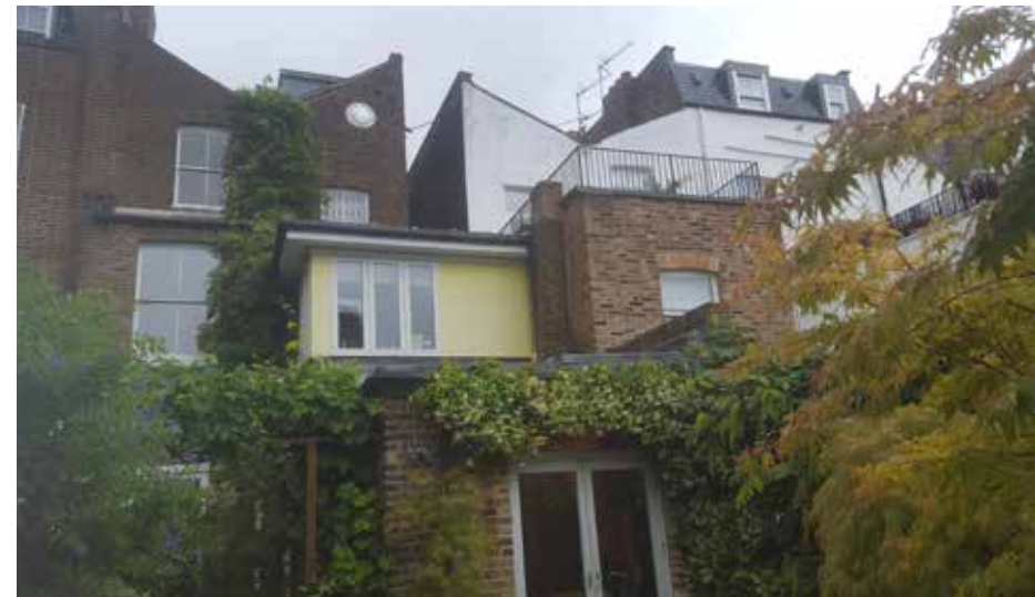
Existing Rear Extension View towards 26 Falkland Road
