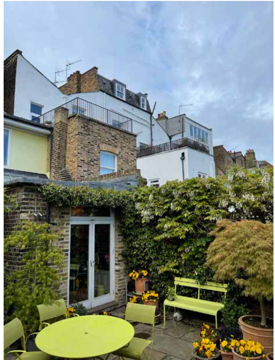
Existing rear elevation -view towards no 26
