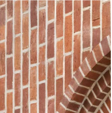
02 Red bricks to Westbere road elevation, with stacked vertical and horizontal brick bonds at ground floor Image to right: Flower Michelin Architects
