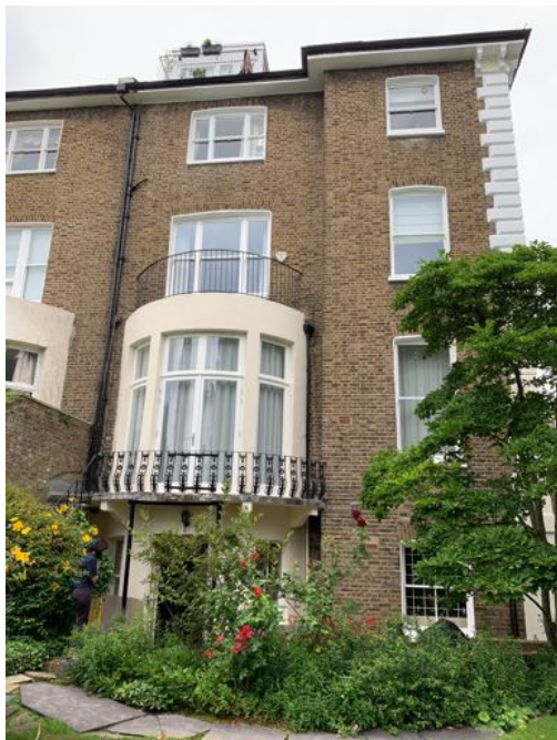
Rear elevation of 8 Belsize Park.
