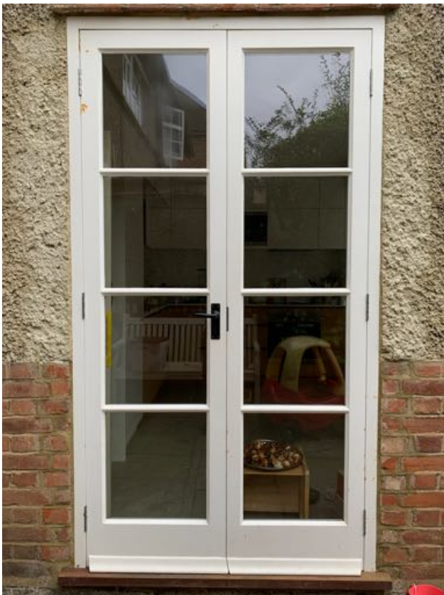
Example of traditional timber-framed, double-glazed, garden doors in a large square pane design.
