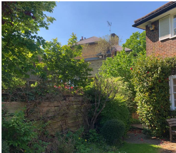
(Photo of the retaining wall, and boundary with the end of 18 Frogmal Way's garden)
