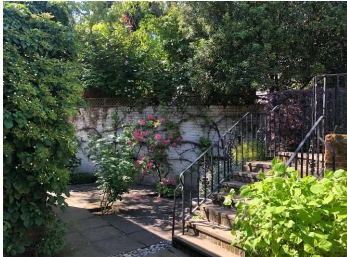
(Photo of the retaining wall, and boundary with the end of 20 Frogmal Way's garden)
