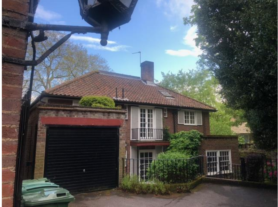
(View of existing front façade with protruding 1.5 storey tall block)
