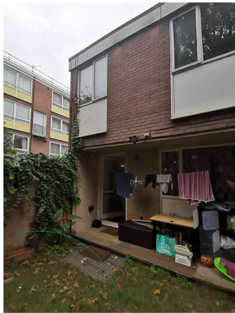
Existing Boundary Brick Wall With Residential Block Clarence Gardens
