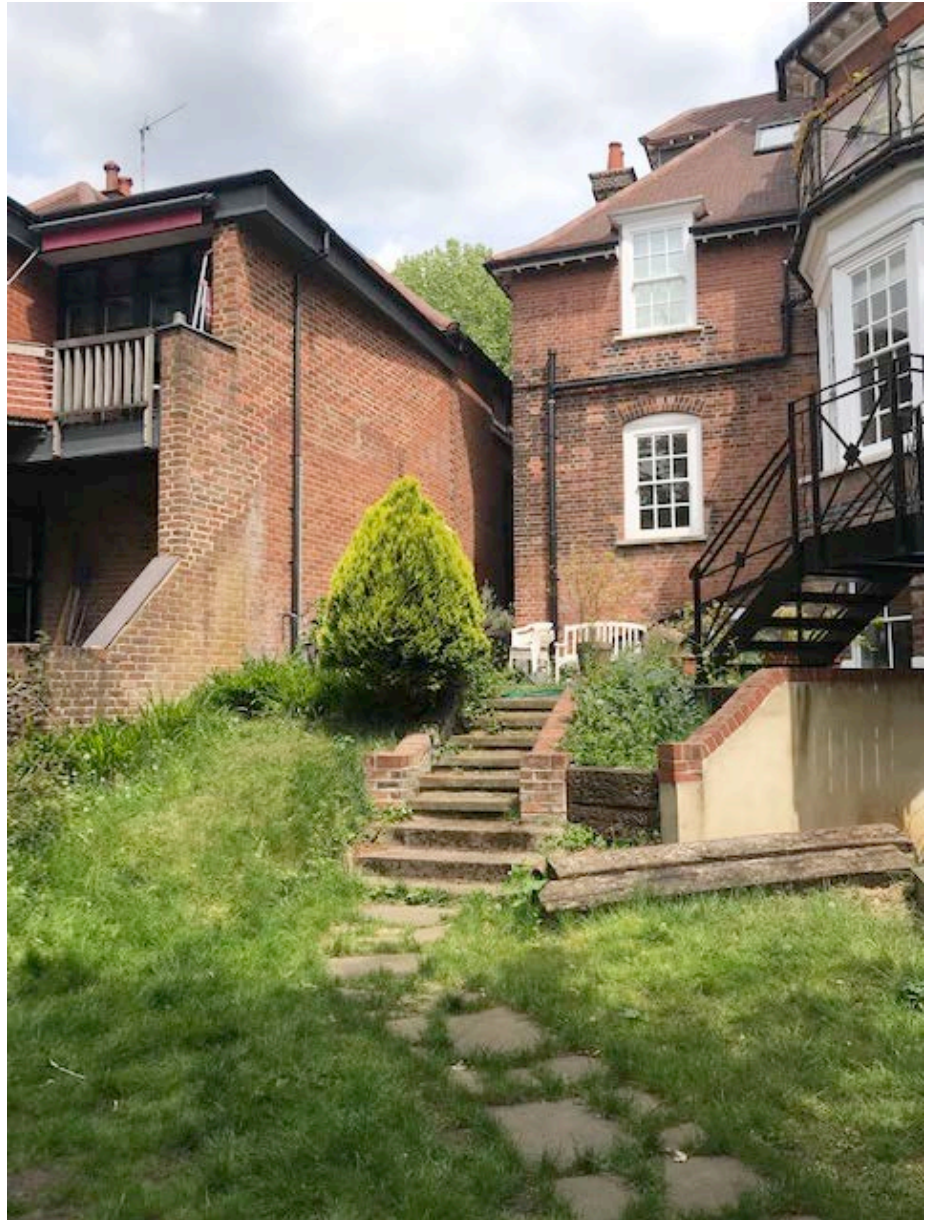
Photo 4: Taken facing east towards number 7 rear elevation and illustrates side access pathway to be used for extraction and delivery of materials (No access for plant or heavy machinery)
