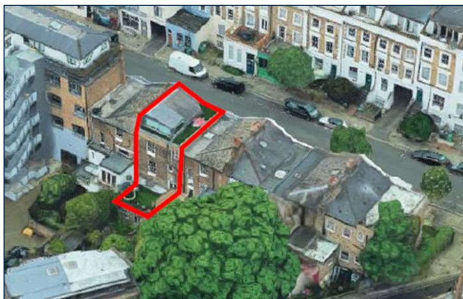
Above- Aerial view of the site showing existing roof extension
