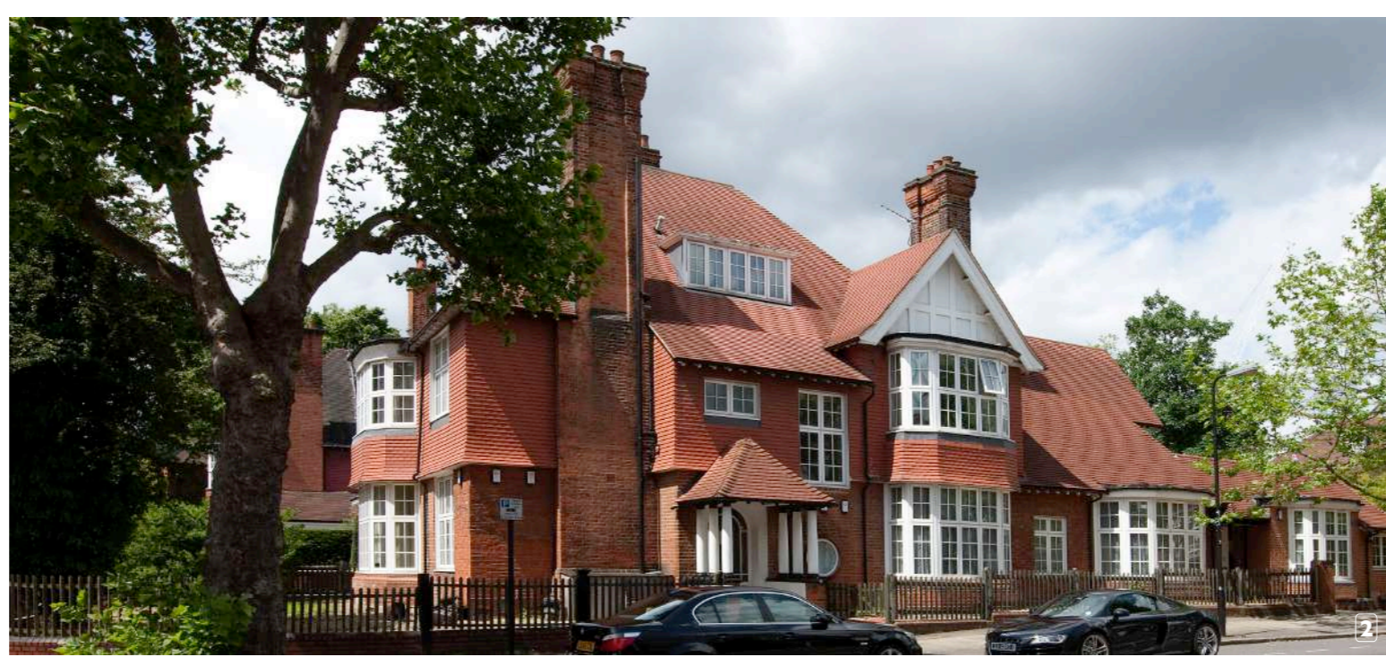
EAST-MAIN FACADE - WADHAM GARDENS
