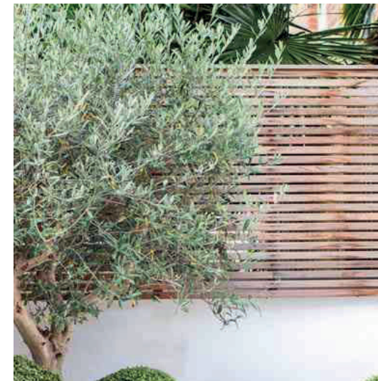
Rear side and back boundary Horizontal timber slates fence on top of white rendered wall
