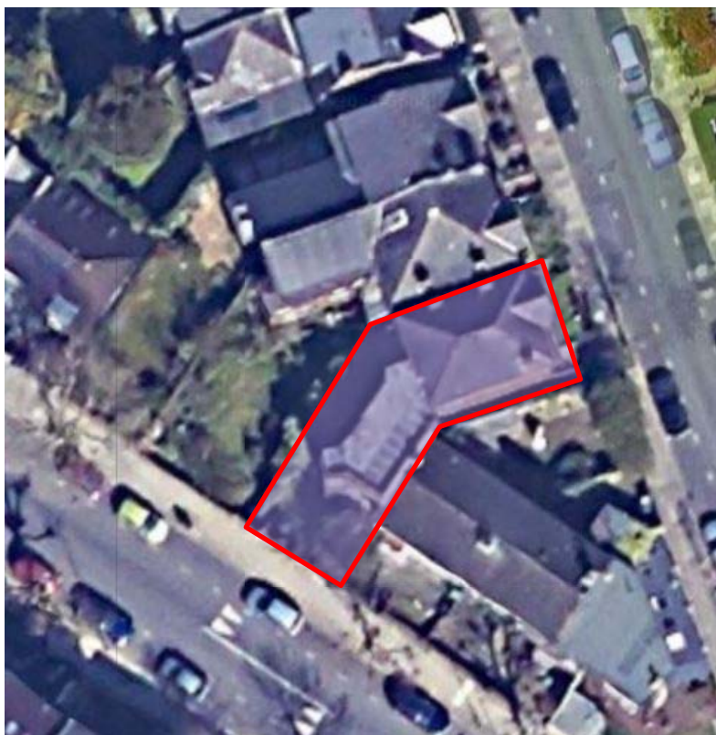
Figure 2: Site view (Google Maps 2021) showing the existing development site (red) in context.
