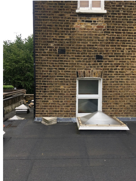
Window to utility cupboard on communal stair landing – note obscured glazing
