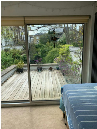
First floor terrace to be retained and railings added for building regulations
