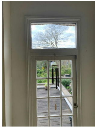
Second floor terrace to be retained and railings added for building regulations
