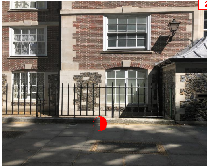
External location for a new 90mm building duct entry to be created into the Lower Ground Comms Room wall from Mecklenburgh Place.
