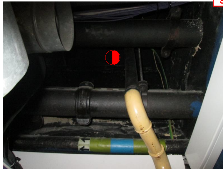
Internal location for a new 90mm building duct entry to be in the Lower Ground Comms Room wall.
