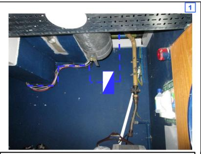
Approx 2m of new VF 12f cable to be installed through new building entry point in Lower Ground Floor Comms Room and will drop down wall to new building flexibility point (BFP).
