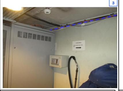
Approx 8m of new VF 12f cable will be installed from new BFP and follow exisisting cables along wall to customer cab where it will terminate in a new Craft Tray (CTP)
