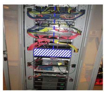
Approx 8m of new VF 12f cable will be installed from new BFP and follow exisisting cables along wall to customer cab where it will terminate in a new Craft Tray (CTP)
