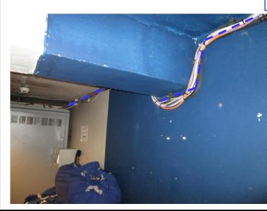
Approx 8m of new VF 12f cable will be installed from new BFP and follow exisisting cables along wall to customer cab where it will terminate in a new Craft Tray (CTP)
