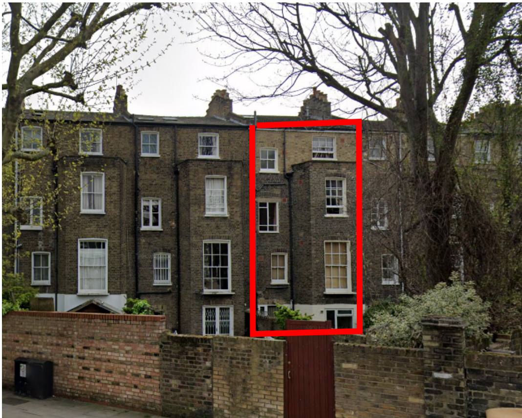
Rear elevation as seen from Canteloves Road
