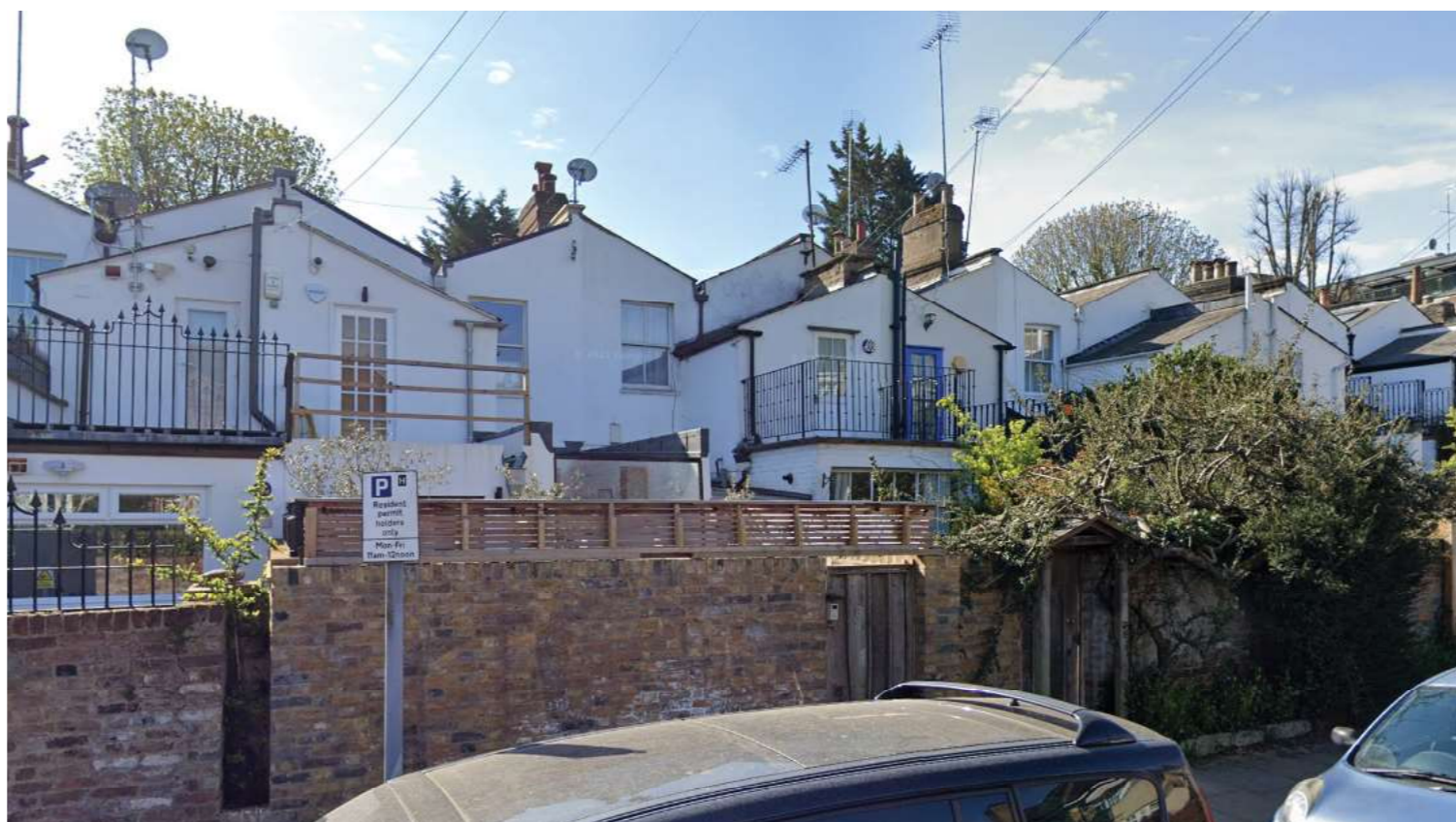
Image 02 . Rear elevation (view from Hampstead Way)
