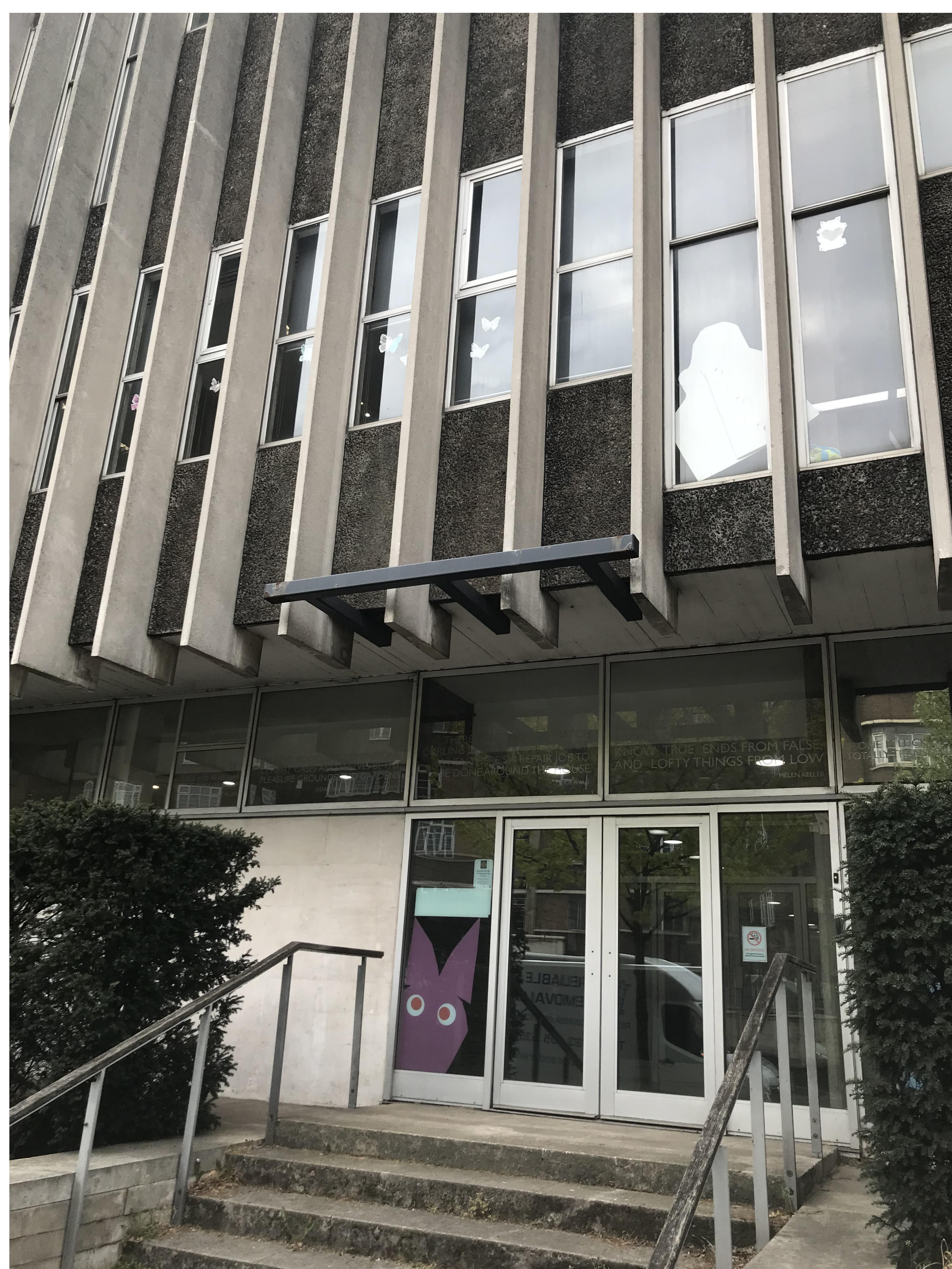
PHOTO SHOWING EXISTING WINDOWS INSITU
