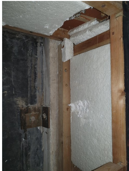
Detail view showing original insulation in the cavity area behind the bookcase
