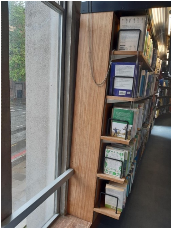
Detail view showing bookcase surround and integrated window board
