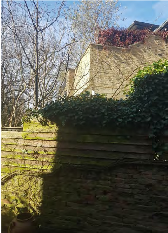
(Photos looking up at 18 Froggnal Way, to show its greater elevation and taller stature)
