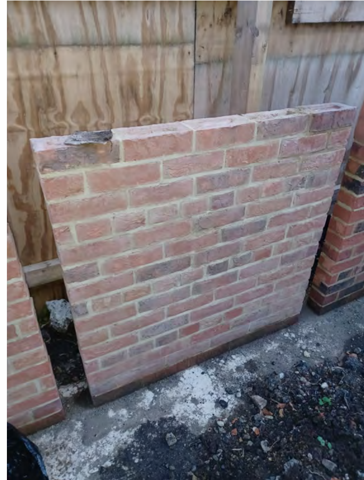
Colorado Red Sample panel built on site
