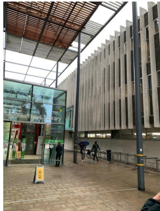
Figure 7 - General view_East elevation
