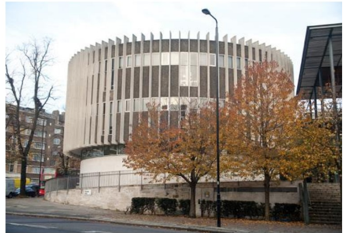
Figure 5 - General view_South elevation
