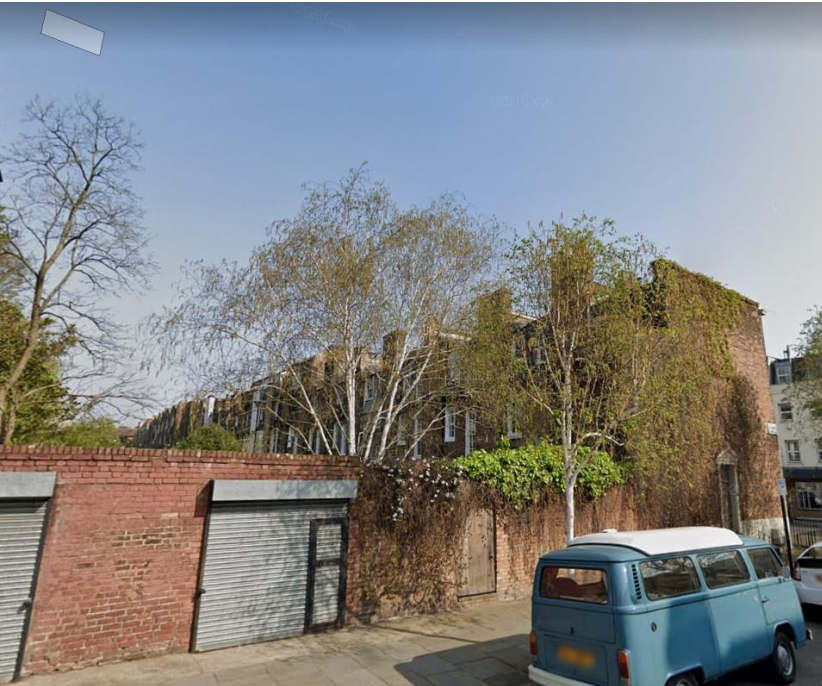
Image 4 (above): View from Mornington Street
