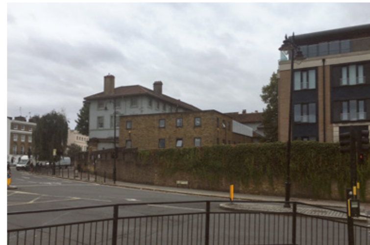
1 Proposed view of the north sandblasted opaque glass boundary on Gloucester Avenue looking south
