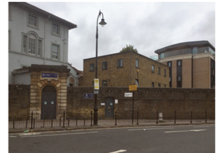
2 Existing view on Gloucester Avenue looking west
