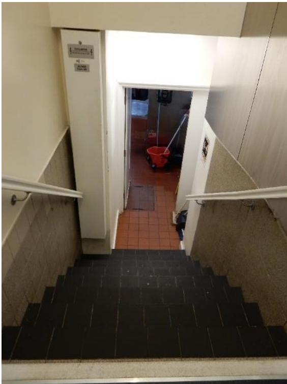
Existing steps from Corridor to Production Kitchen
