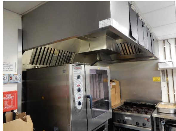
Existing Pastry Kitchen looking NE
