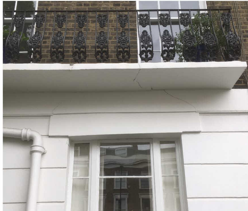
Figure 1 Ground Floor Window
