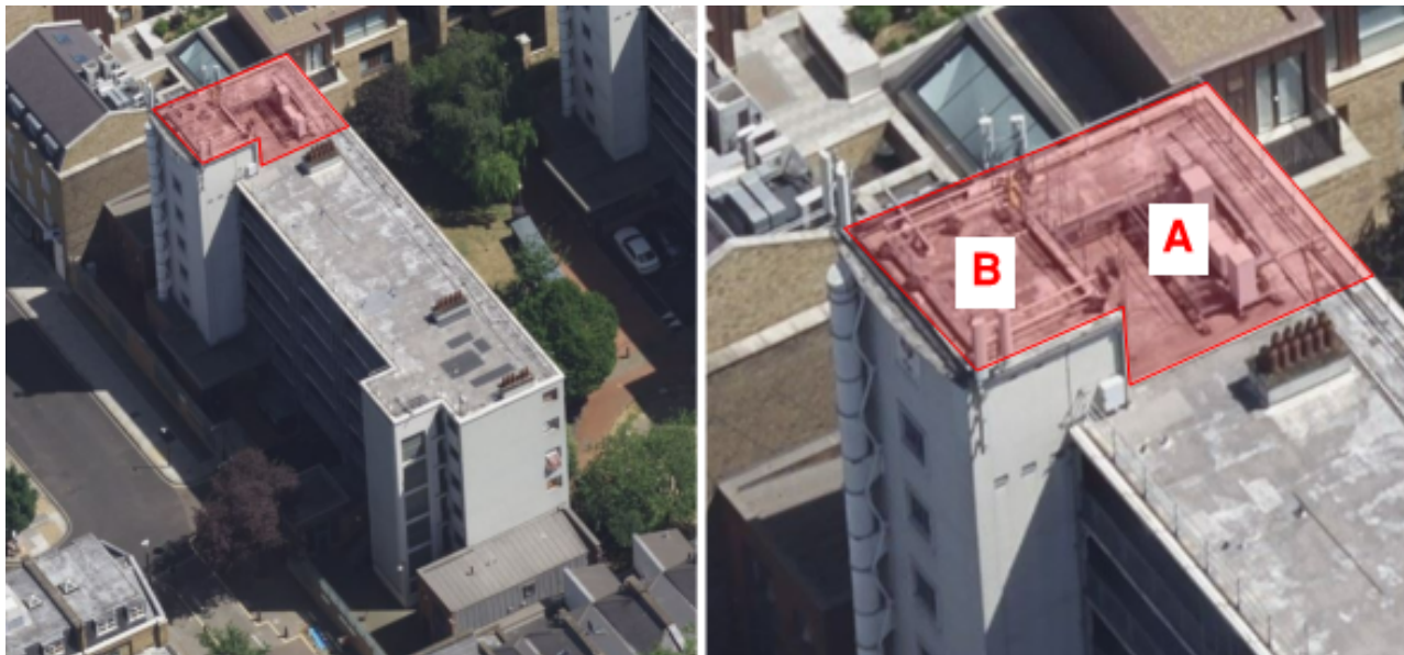
Images 1 and 2 – aerial views showing relevant roof areas of building
