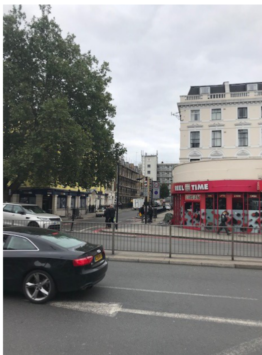
Existing equipment (view from north, King's Cross Station, Euston Road)
