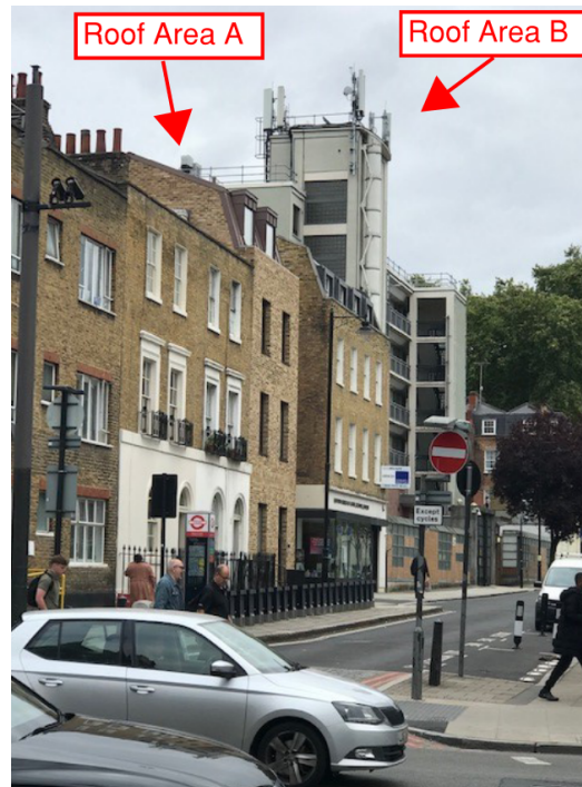
Existing equipment (view from east, Gray's Inn Road)
