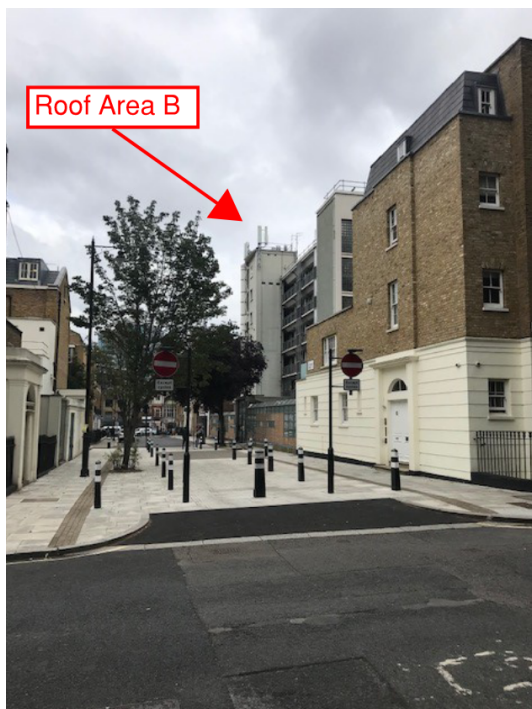
Existing equipment (view from west, Argyle Square)
