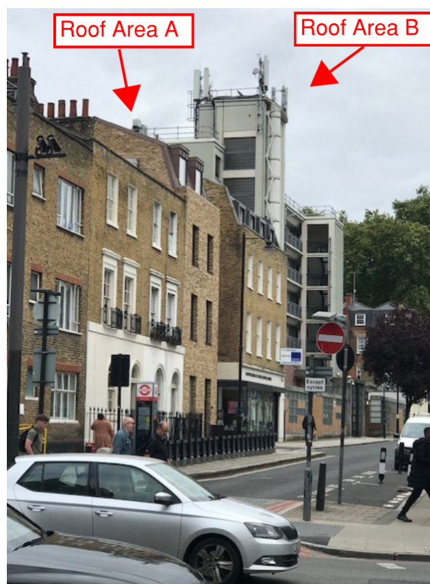
Image 4 – existing equipment (view from east, Gray's Inn Road)
