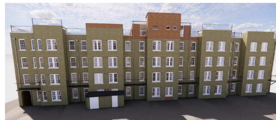
EXISTING REAR FACADE
