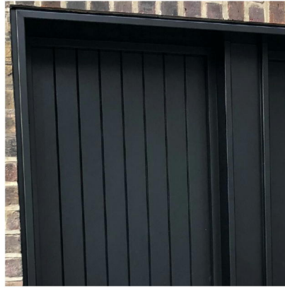
Figure 2 Proposed scheme (ref: 2021/3029/P) with polyester powder coated, aluminium-clad front door and gate; seams at shorter intervals (approx. 100mm).
