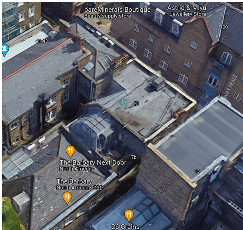
21 – Site of proposed roof top plant, raised parapet wall and rear kitchen extract duct
