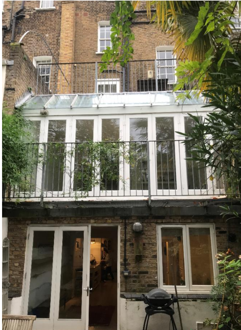
Plate 2: Rear (east) elevation. This photograph clearly shows the 1990s rear extension; balcony and railings to ground and railings to first floor
