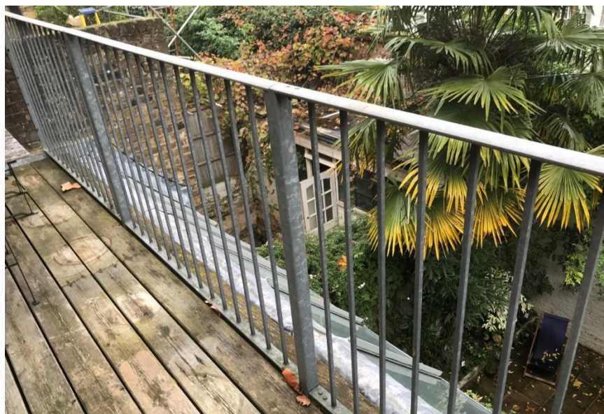
Plate 4: First floor railings (to be removed and replaced with glazed panels)
