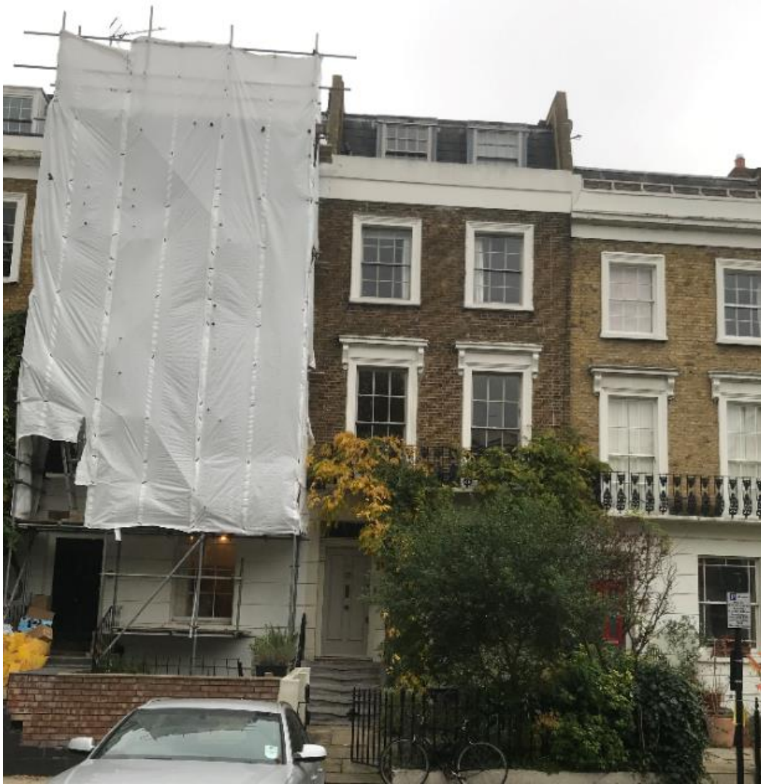
Plate 1: Principal façade. West elevation.
