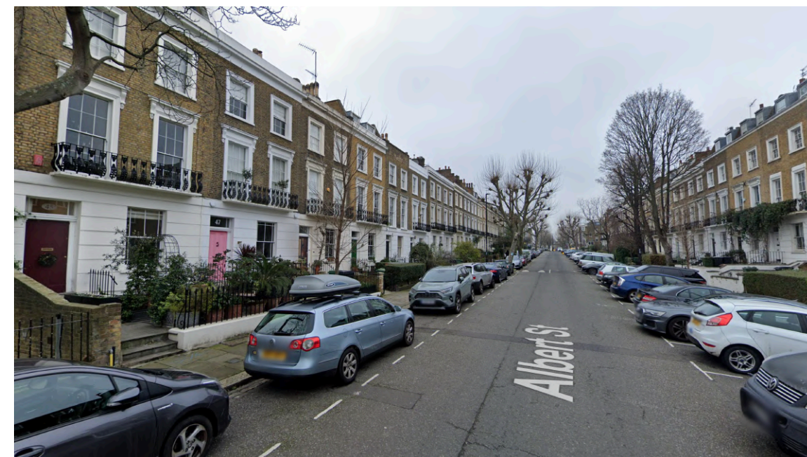
View looking towards the North of Albert Street
