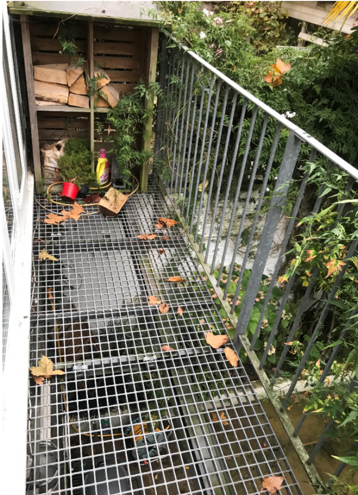
Non-original steel rear balcony
