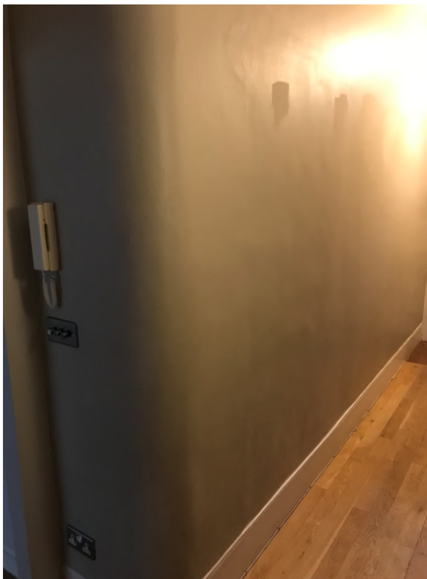
Ground floor historic door position
