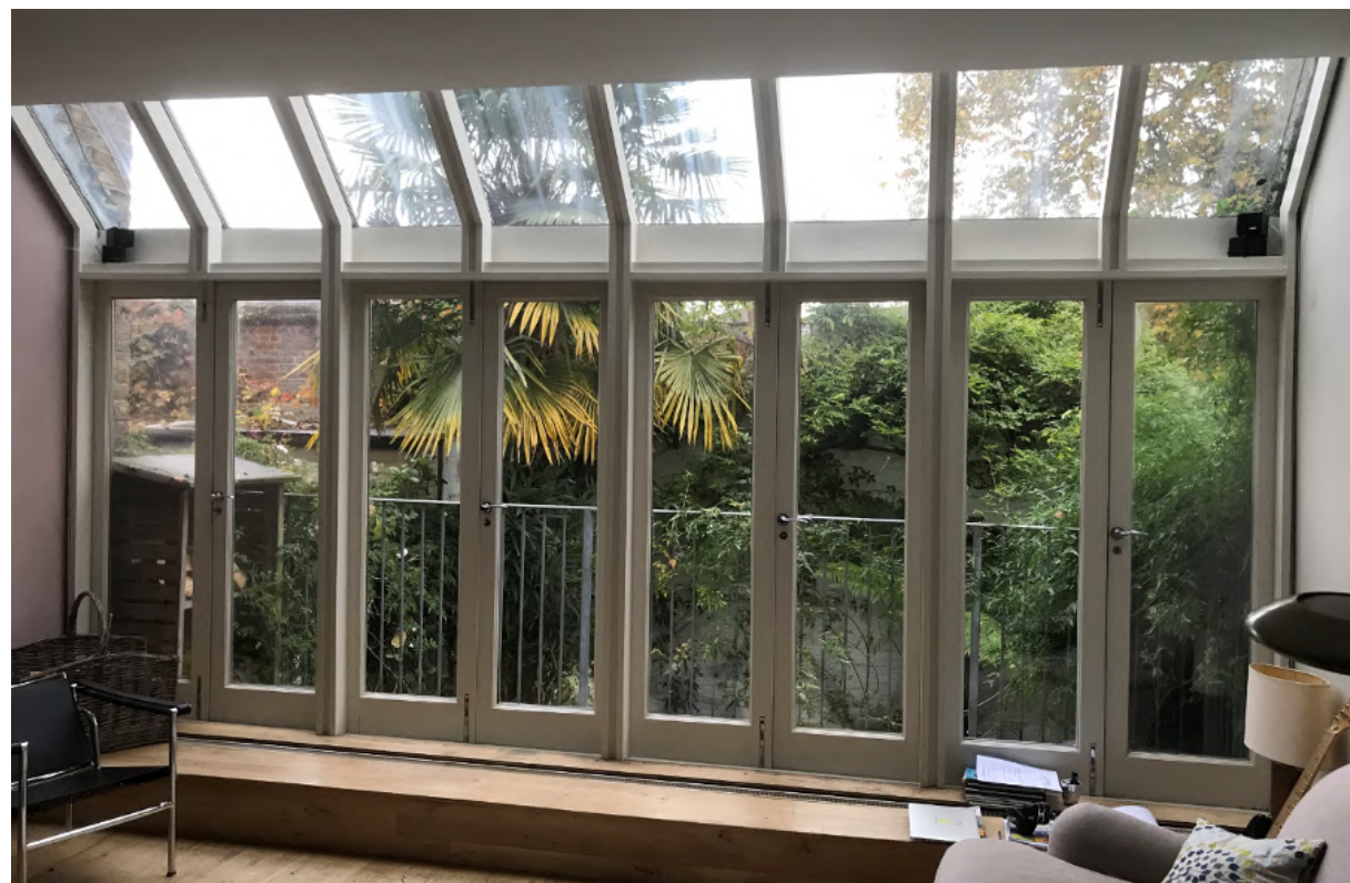
Existing ground floor rear doors
