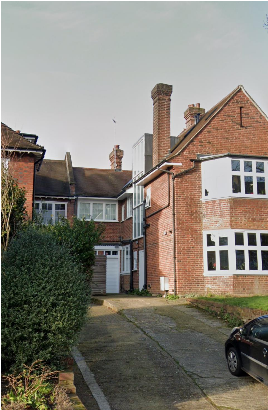
Photo 4: No.78 Lawn Road – Side Dormer
