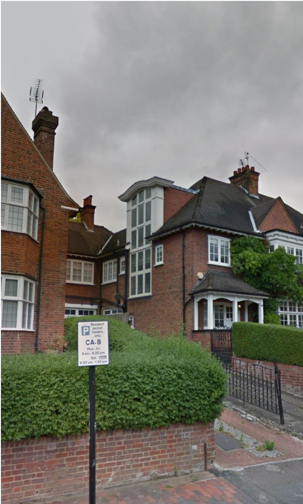
Photo 6: No.80 Lawn Road – Side Dormer
