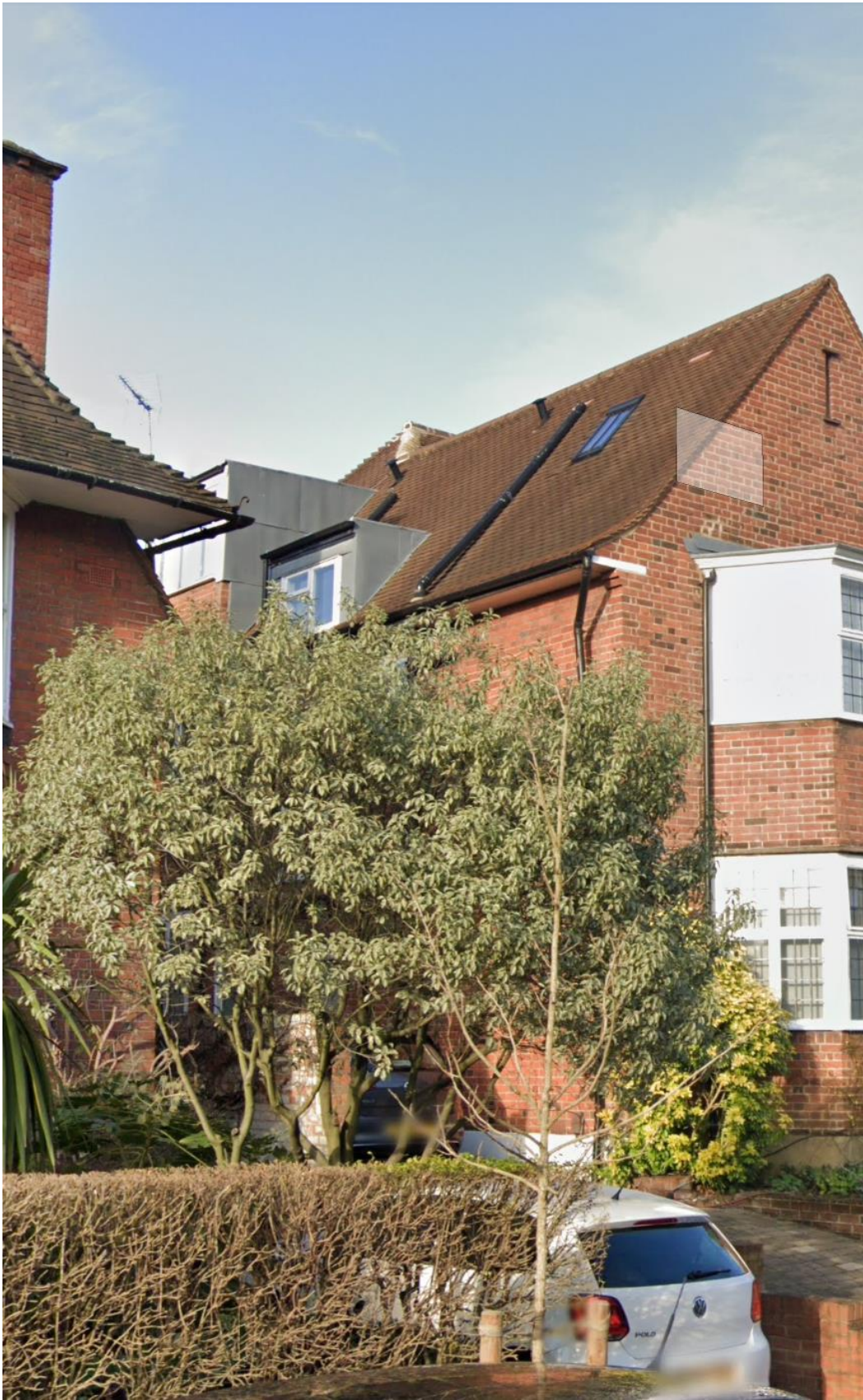
Photo 8: No.82 Lawn Road – Side Dormer
