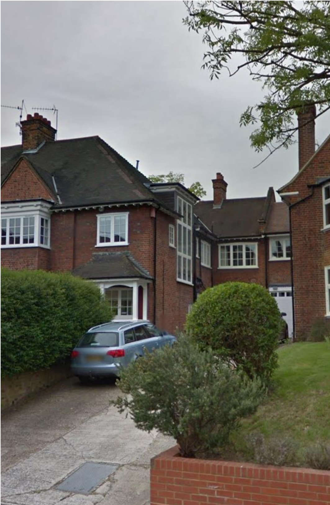
Photo 5: No.79 Lawn Road – Side Dormer
