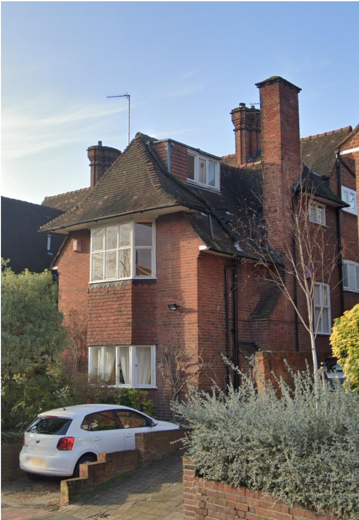
Photo 9: No.83 Lawn Road – Side Dormer
