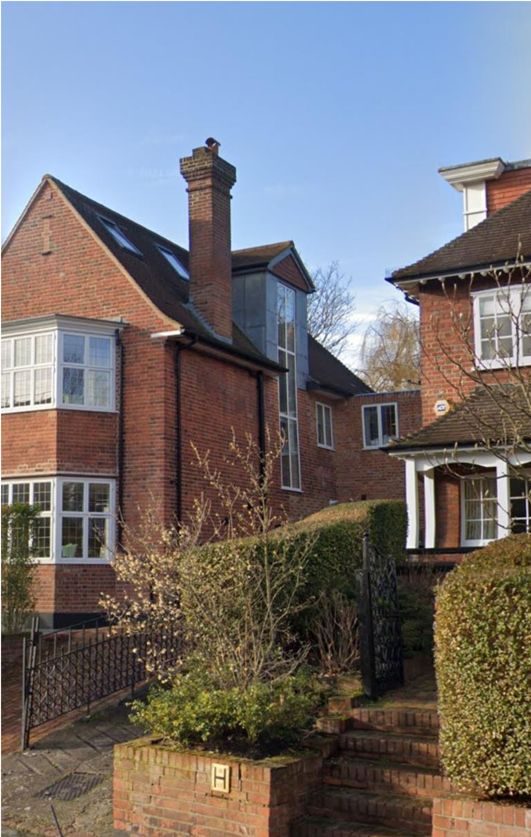
Photo 7: No.81 Lawn Road – Side Dormer
