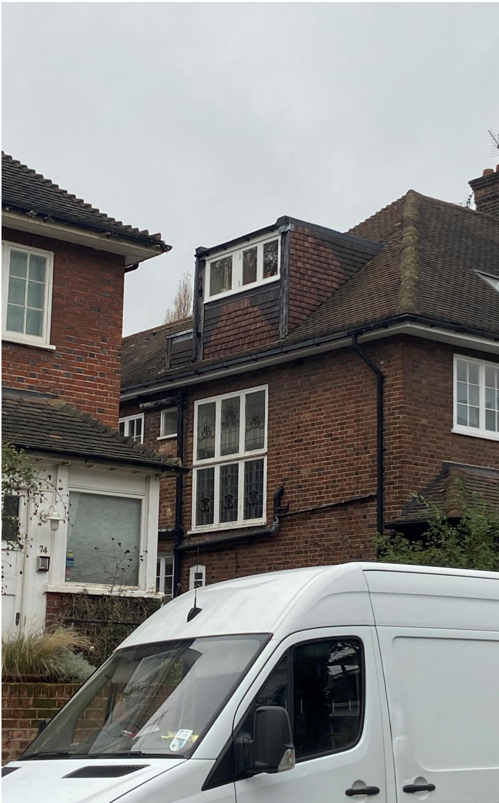
Photo 2: No.73 Lawn Road - Side Dormer
