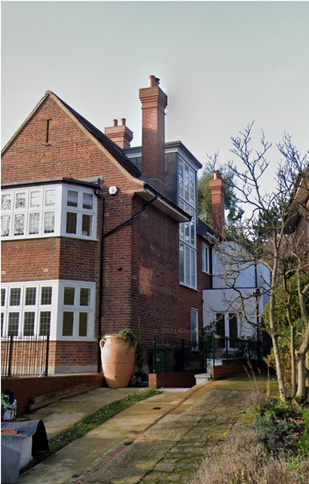
Photo 3: No.77 Lawn Road – Side Dormer
