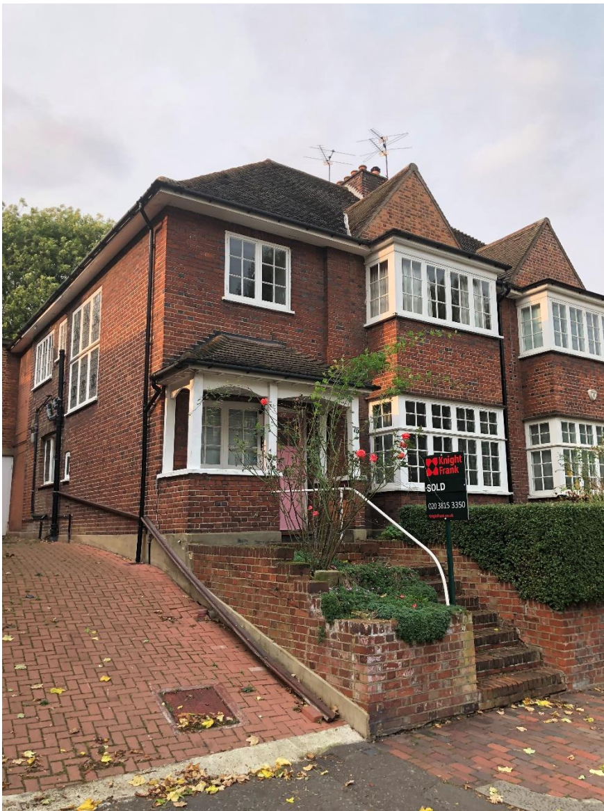
Photo 1: No.75 Lawn Road - Street elevation (looking West)
