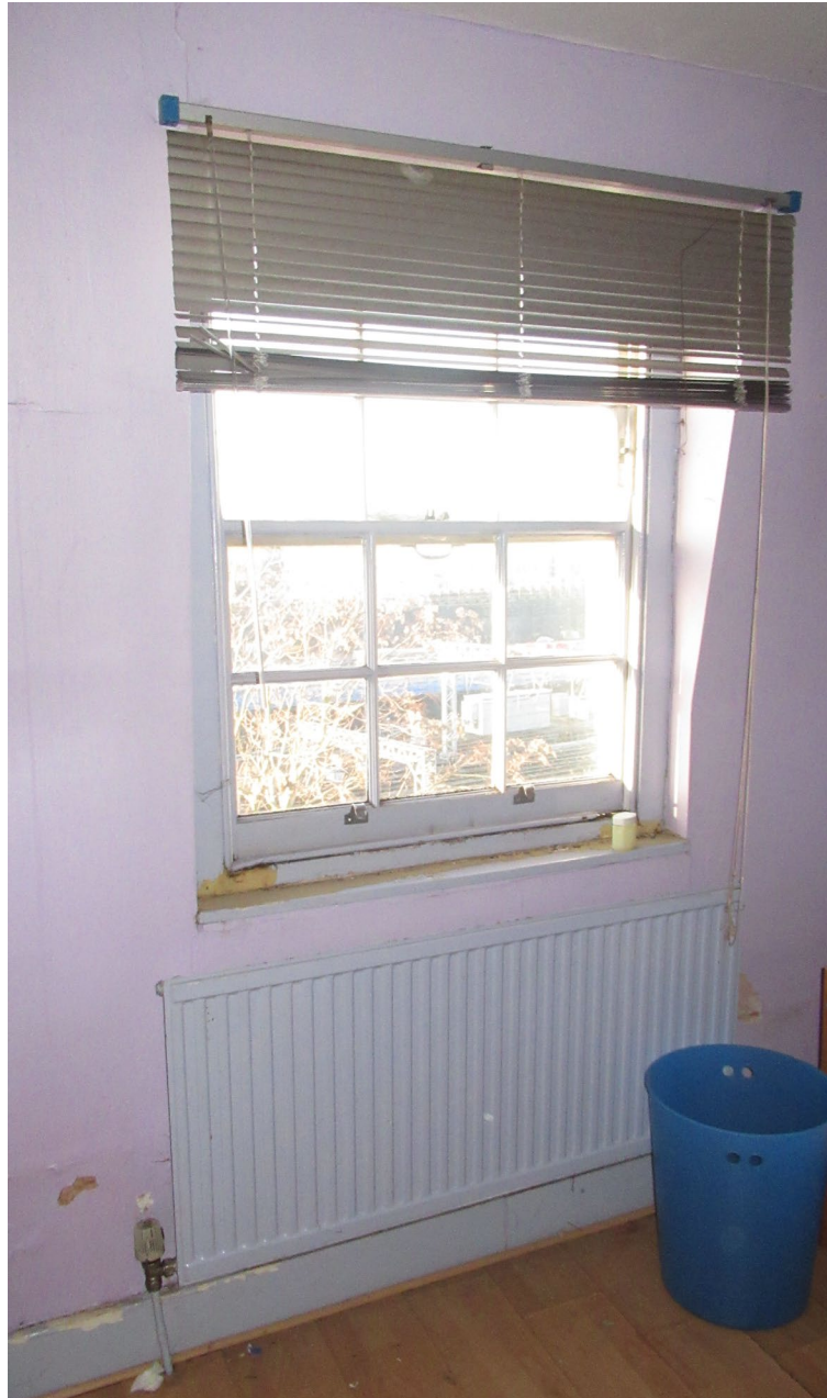
Figure 9: Internal view of window at third floor
