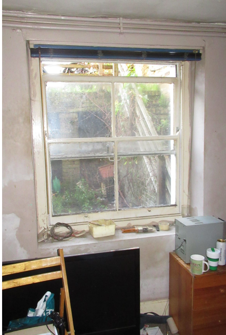
Figure 7: Internal view of window at basement level
