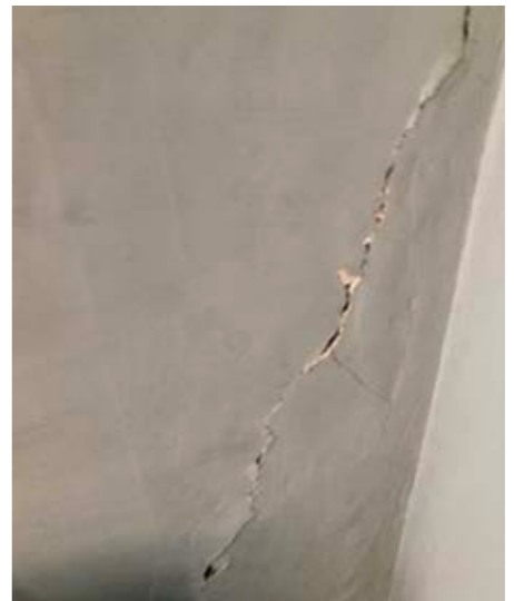
Cracked plaster to rear wall
