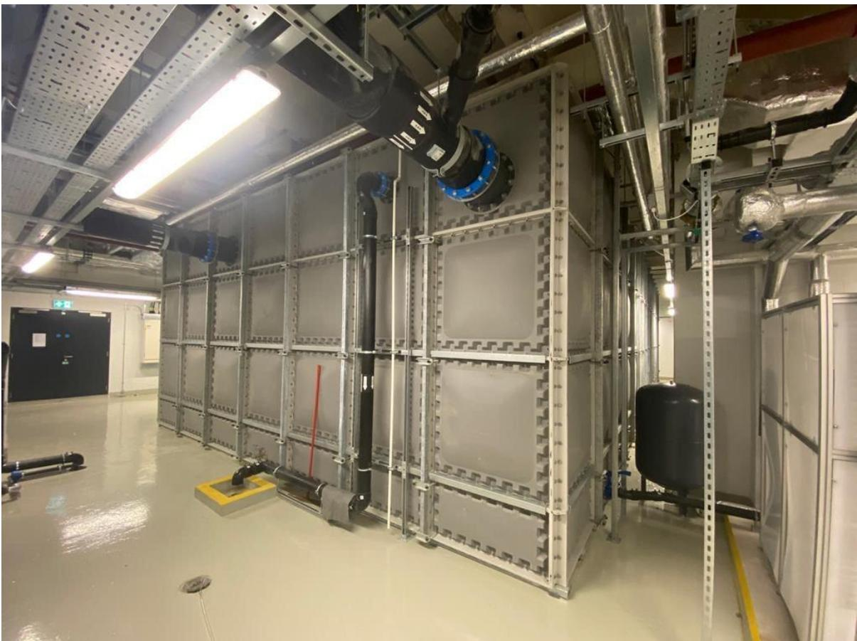
**PHOTOGRAPHS OF THE INSTALLED ATTENUATION TANK IN SITU WITHIN 1 TRITON SQUARE, AS SHOWN ON AS BUILT DRAWING NO. 4185-03-ATT-GW**
