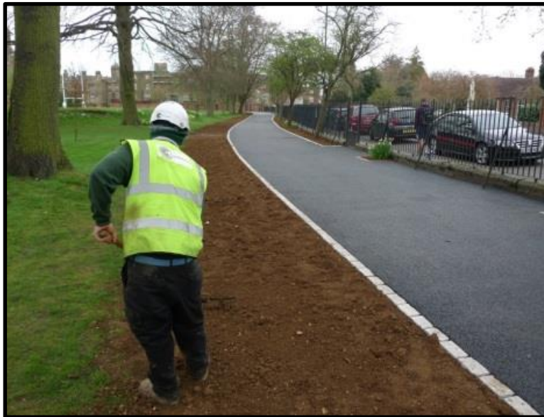
Fig 9 – All 'making good' topsoil will be BS3882 compliant and raked out by hand to no greater depth than 100mm
