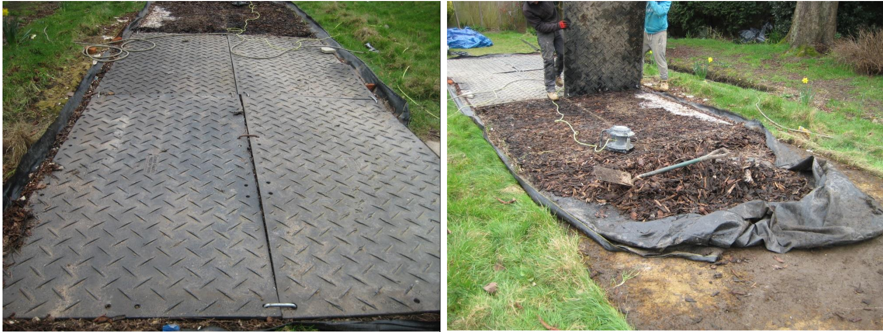
Fig 8 – Temporary ground protection is an effective way of allowing access through the RPA of retained trees. It must be installed prior to any on site activity and maintained for the duration of all works to be effective. Above left Tamla Trees project ground protection in place and above right being removed following the completion of site works. (Note: depending on the length of time it is in place it will adversely affect underlying grass ground cover which will need reseeded/ turfed accordingly)
