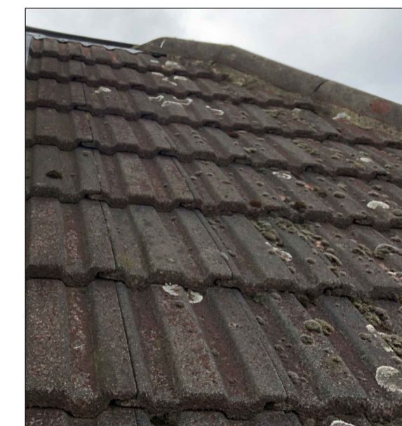
Top Image: Existing GF Timber frame glazed Doors as viewed internally from the kitchen area Bottom Image: Existing roof tiles
