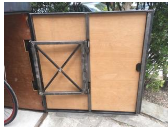
Heavy duty hidden double hinging and ply panel linings
