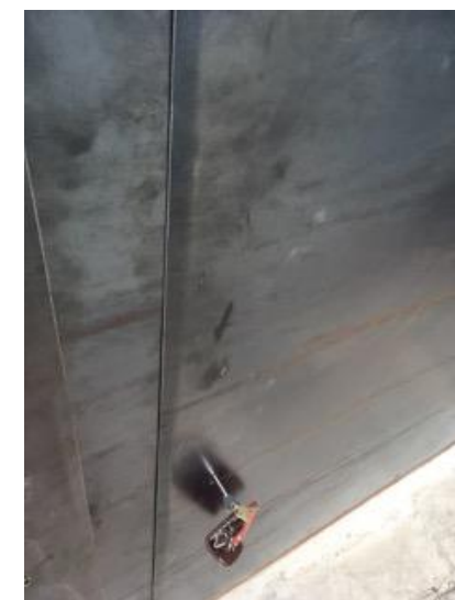
Flush finish doors with 5-lever mortice key locking.
