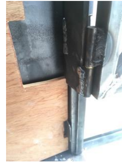
Heavy duty hidden double hinges with anti-jemmy detailing
