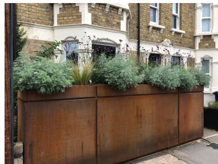
Bikebox is made of 2mm mild steel, attached to concrete & steel base constructed in situ.
