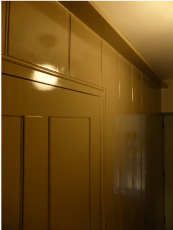
Fig. 2 Finished T&G paneling with shelf close to ceiling level.
