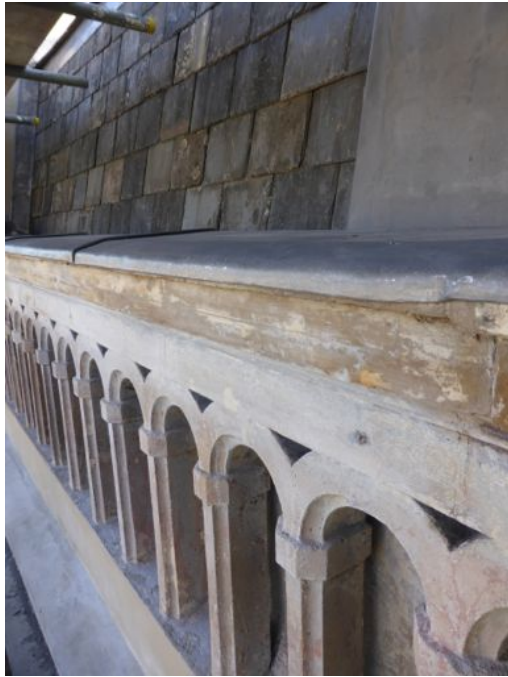
Fig. 14 lead cloak to parapet as installed
