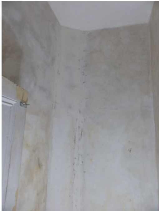
Fig. 5 Boxed in waste pipe to cloakroom (plastered awaiting paint finish).
