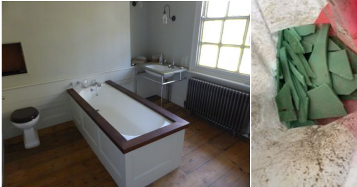
Figs. 6, 7 Master bathroom with shattered 'Vitrolite' splashback.
