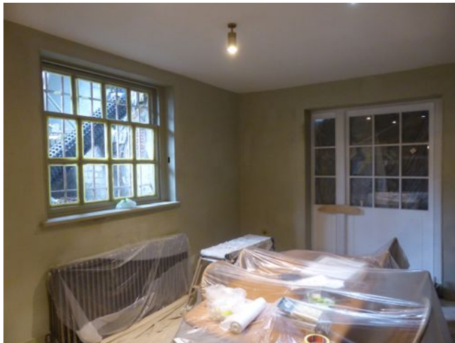
Fig. 1 Dining room interior showing revised glazed door proportioned to the original sash windows.
