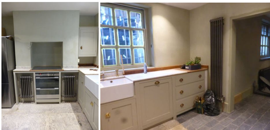
Figs. 3,4 Finished kitchen units with mahogany splashbacks and revised radiator locations
