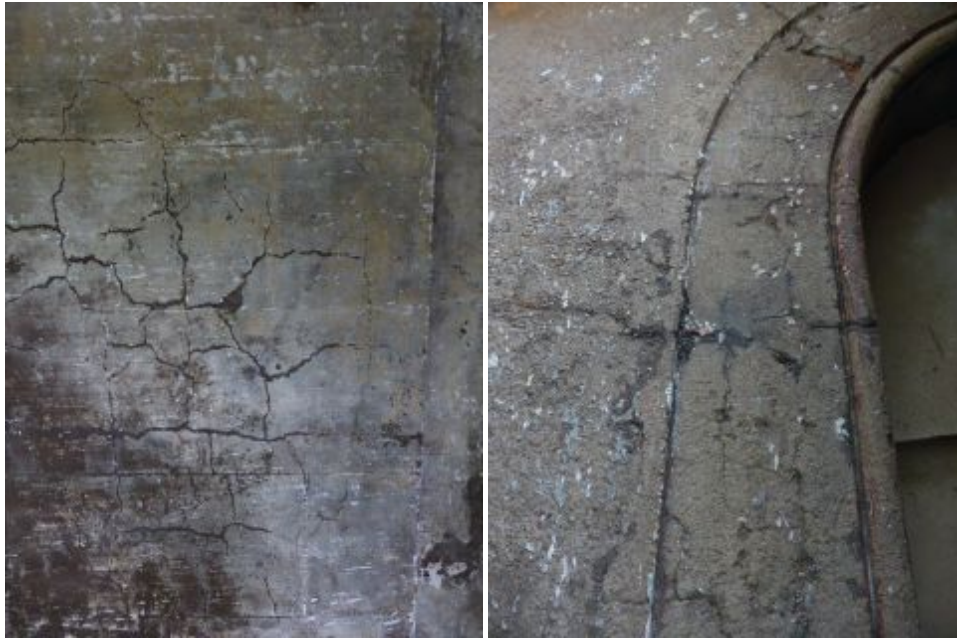
Figs. 11, 12 following Thermatech paint removal
