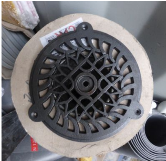
Fig. 10 cast iron grille prior to fitting, to be set flush to the Roman cement render, painted to match walls.
