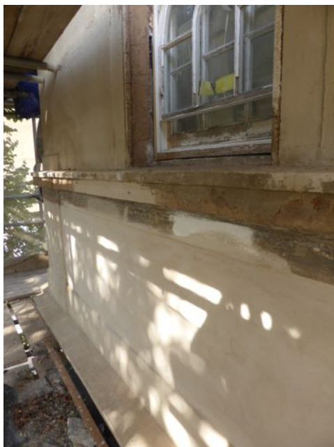
Fig. 13 skim coating in progress, mouldings retained as found.
