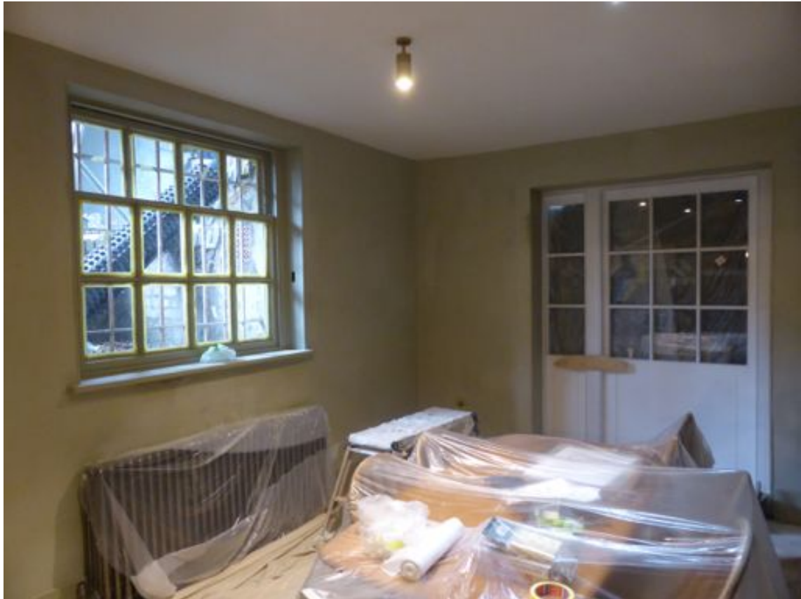
Fig. 5 North door re-proportioned to suit the original sash windows.
