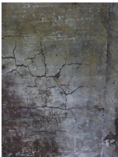
Fig. 10 surface fissures at first floor level
