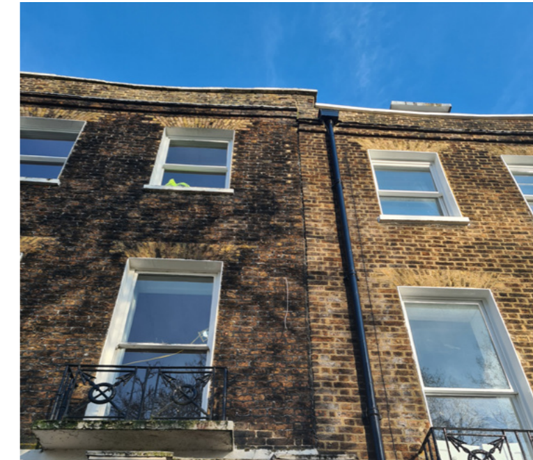
Images of exterior and existing pointing conditions - poor, weathered and dirty.
