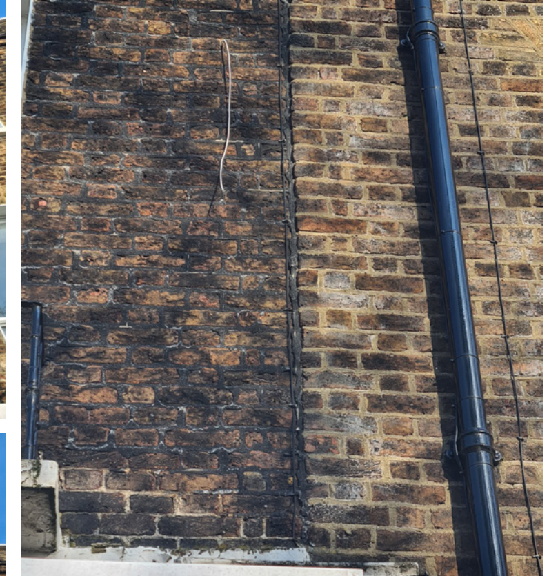
Images of exterior and existing pointing conditions - poor, weathered and dirty.
