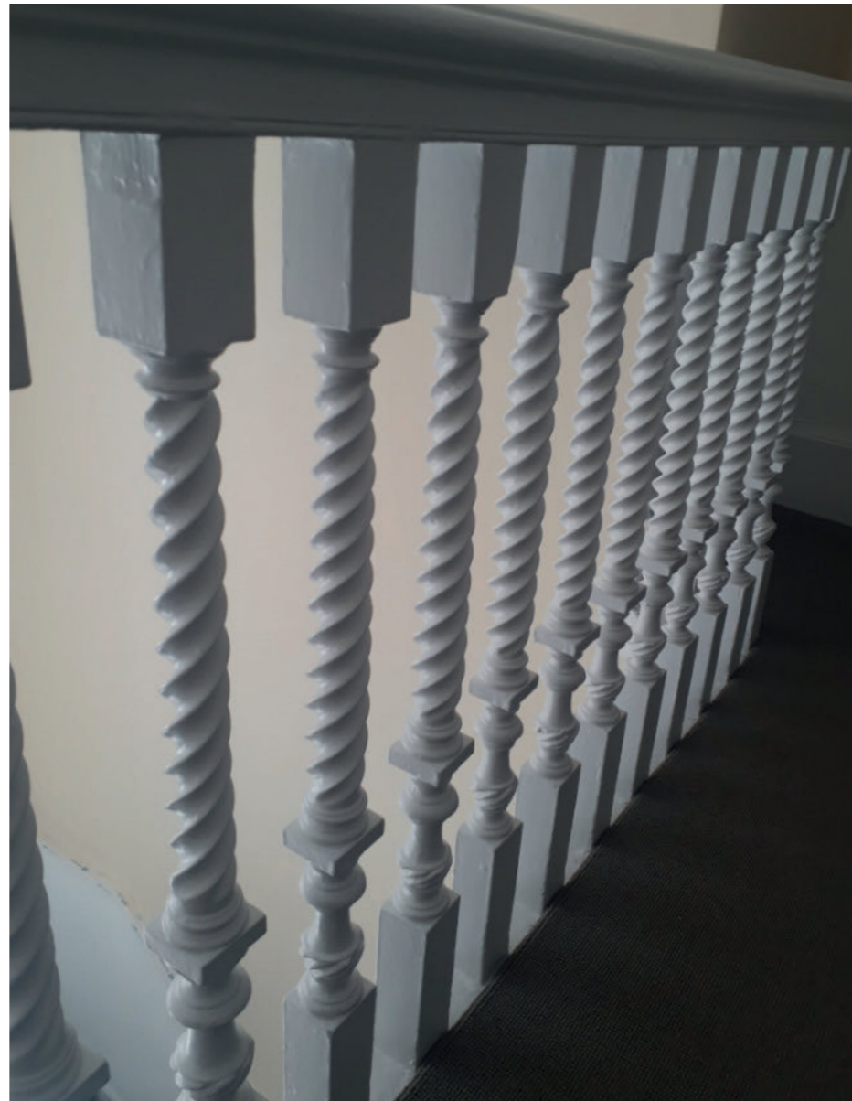
Figure 3.10 Stair balustrades at upper level
