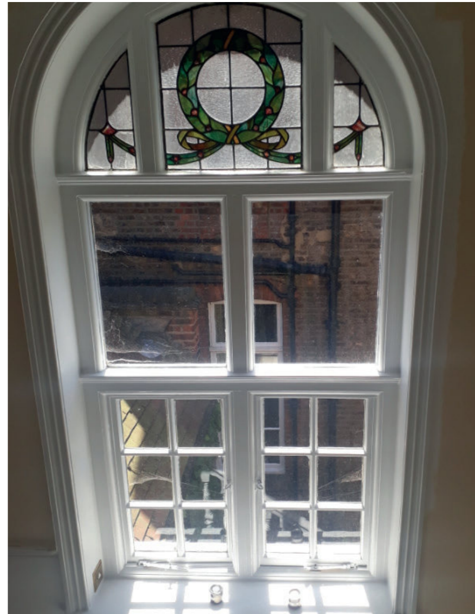
Figure 3.14 Stairwell window, the glazing bars matching designs shown in Figure 3.8
