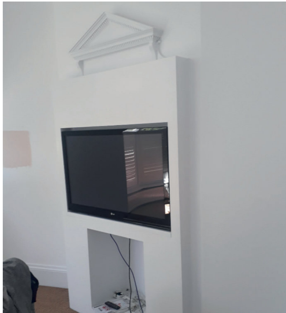
Figure 4.1 Unsympathetic alterations to where a fireplace would have originally been situated
