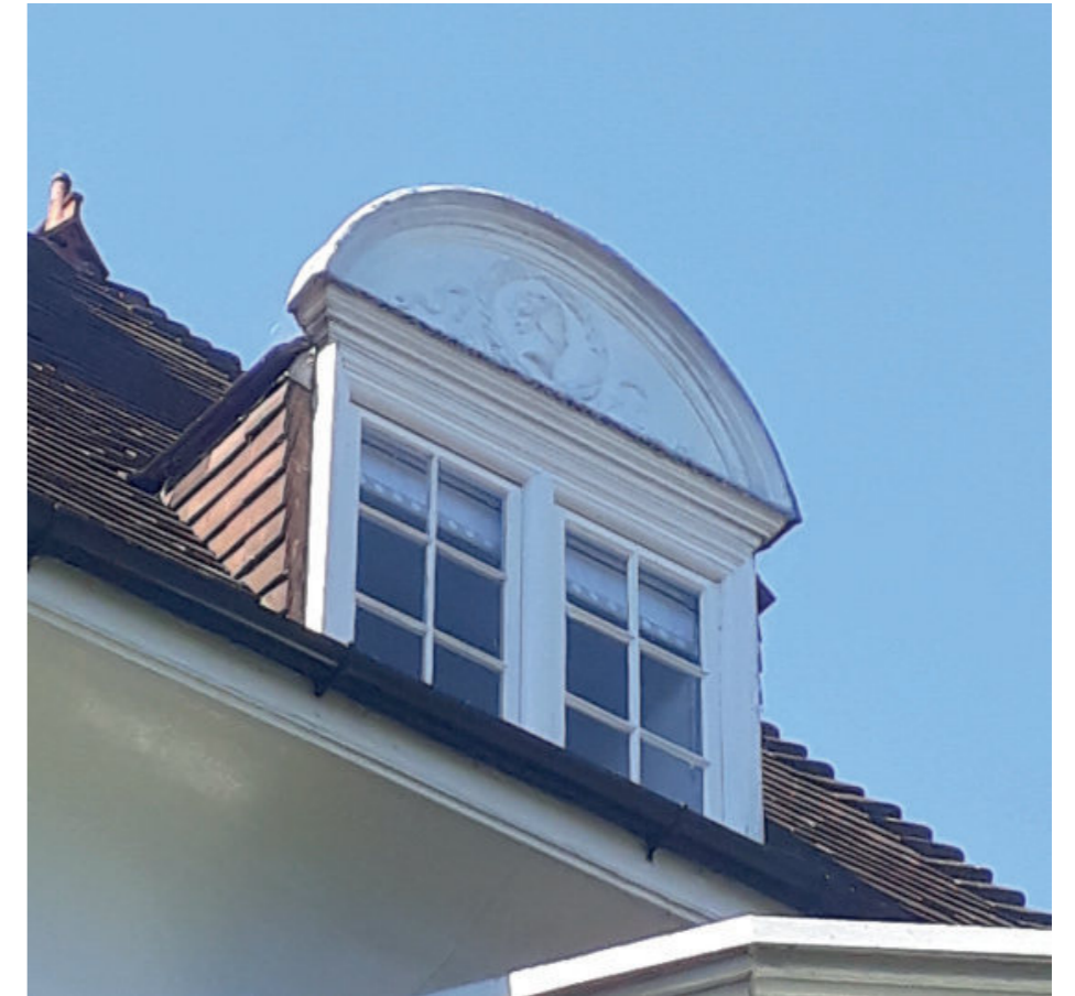
Figure 3.15 Plaster wreath in Classical style on front elevation of building
